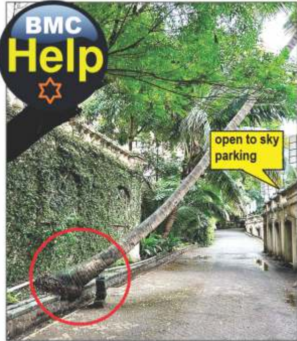
The about-to-fall coconut tree at Galleria Hiranandani resting precariously on bricks. Need to be cut immediately to prevent any accident
